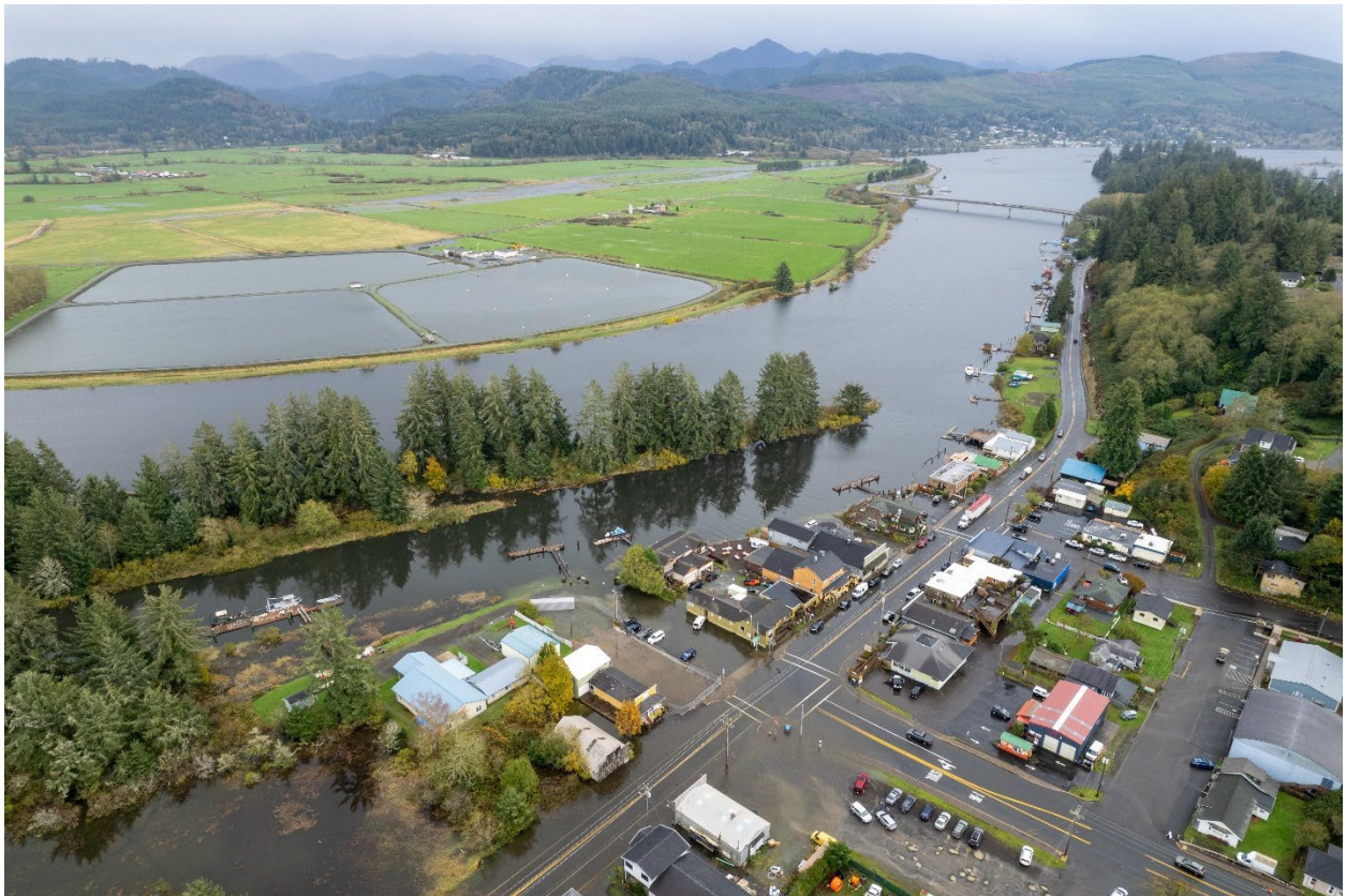
Downtown Nehalem and Nehalem Bay Wastewater Agency, Nehalem Bay, 2021. Photo courtesy of Tyler Sloan.
