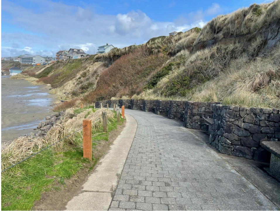
Photo 5: Access Site 5 – Paved Walkway Adjacent to Steep Slope
