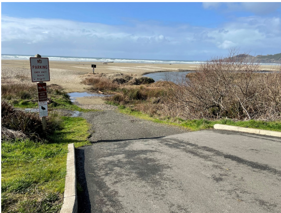
Photo 8: Access Site 8 – Ramp and Creek Crossing
