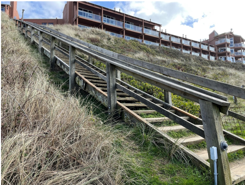
Photo 4: Access Site 4 – Access Structure on Steep Slope
