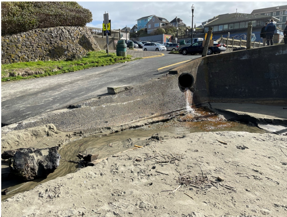
Photo 6: Access Site 6 – Ramp to Beach Adjacent to Retaining Walls
