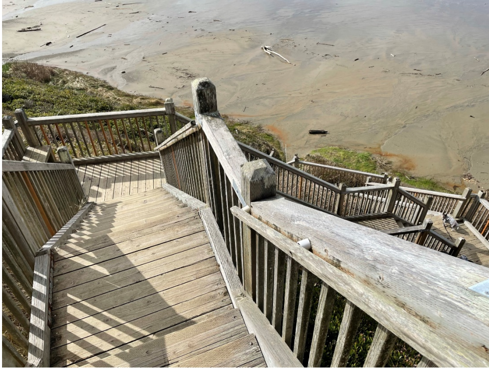
Photo 3: Access Site 3 – Access Structure on Steep Slope
