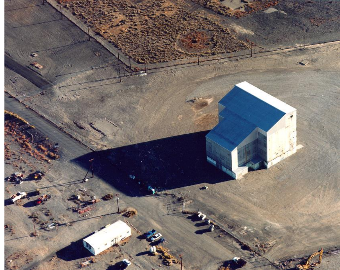
C Reactor in Interim Safe Storage
