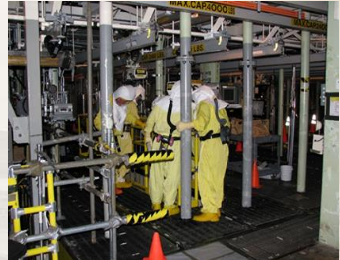
Workers on grating above K West Basin
