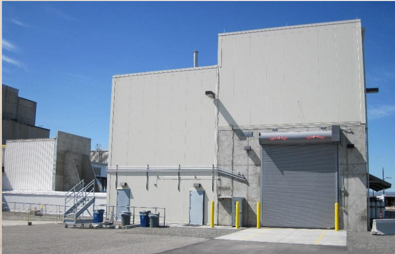
Outside K West Annex
