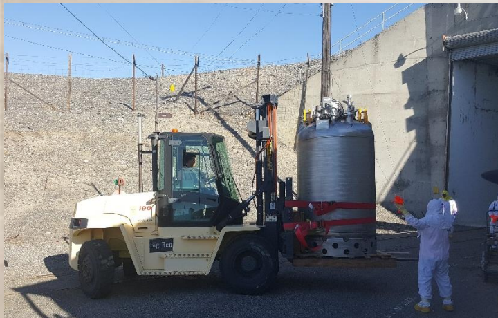
Workers delivering STSC to T Plant
