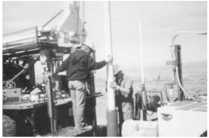
Installation of groundwater monitoring well at the Hanford Site
