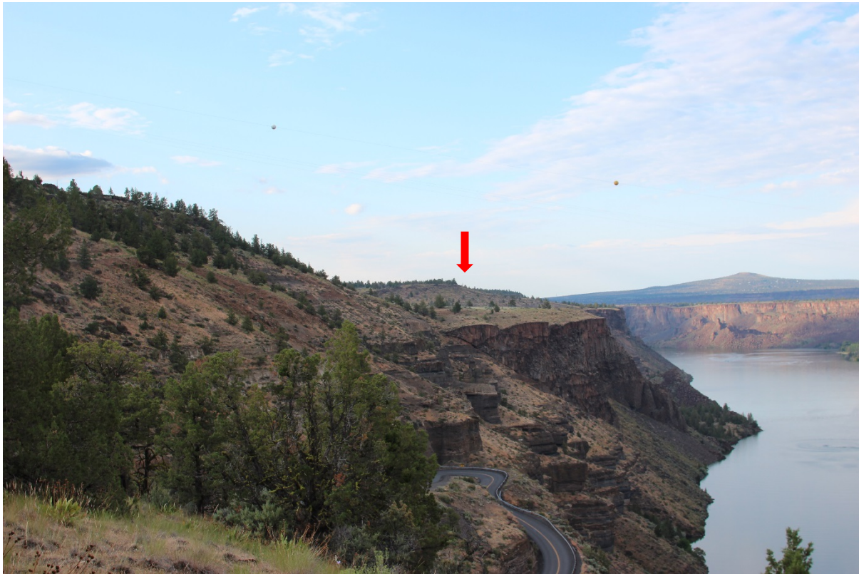
Photograph R-12 – From Photo Survey Point R-12 on Figure R-2: View from a portion of the Deschutes Canyon – Steelhead Falls Wilderness Study Area accessible from the northbound shoulder of SW Jordan Road and adjacent to the Deschutes River’s inlet to Lake Billy Chinook heading approximately 20° N toward the Facility site boundary. (The red arrow indicates the approximate location of the Facility site about 9.9 miles north of Photo Survey Point R-12.)
