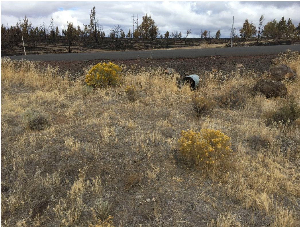
Photograph 4: PP1 – Facing North Elk Drive Roadway culvert
