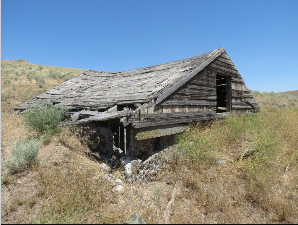
Photograph 2. Pendleton Ranches Sheep Camp Cistern, View Northeast, 7/7/17
