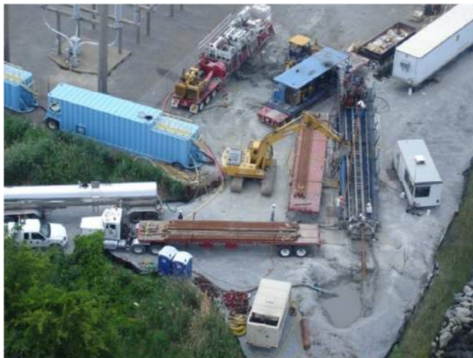
Figure 7: Typical HDD Setup (Lower Voltage Example)
