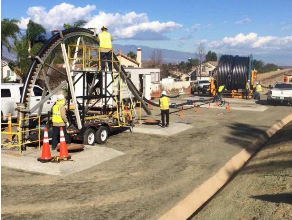
Figure 4: Typical Cable Pulling Setup
