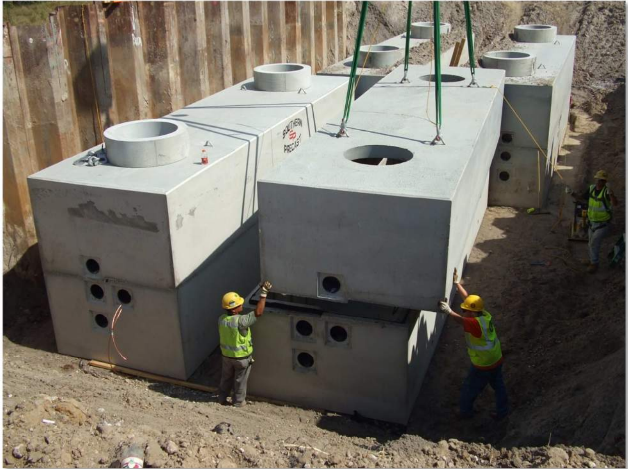
Figure 3: Typical Splicing Vault Installation (lower voltage example)
