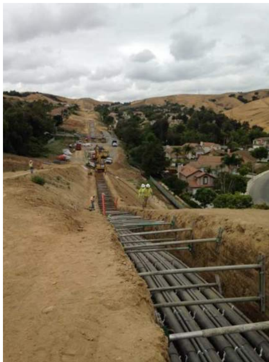
Figure 5: Typical Trench Excavation (Single Trench Only)
