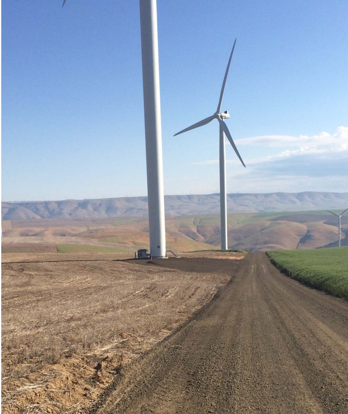
Photo 1 – Example of a constructed crane pad at Turbine #61.
