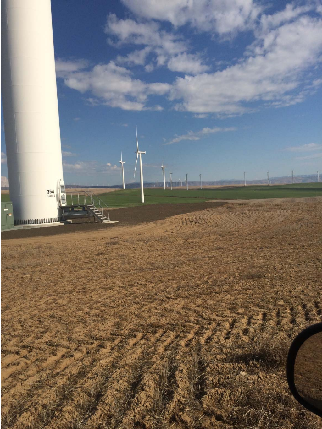
Photo 3 – Example of a constructed crane pad at Turbine #354.
