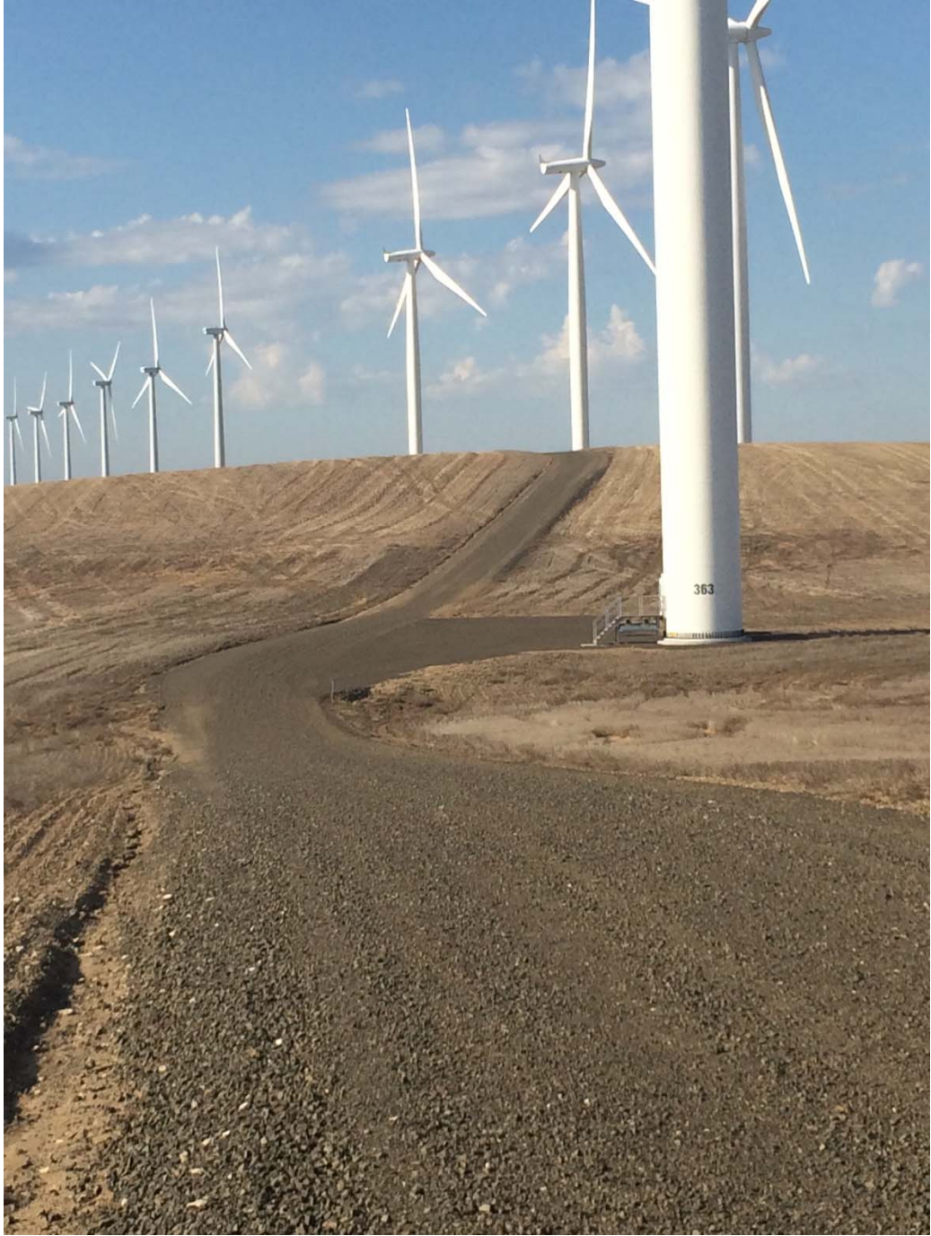
Photo 2 – Example of a constructed crane pad at Turbine #363.
