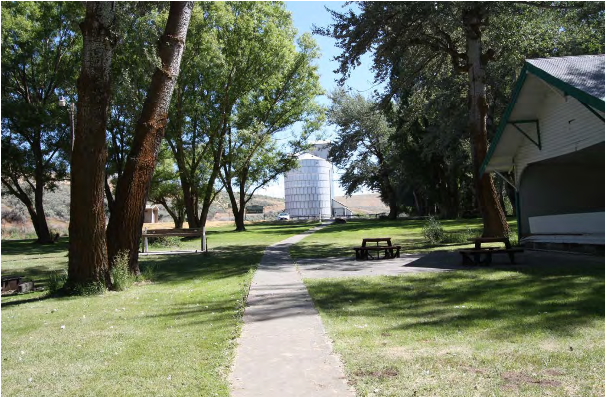
Photo 10. View from within park looking back toward Project on adjacent ridgeline. Looking S. 6/15/2018.
