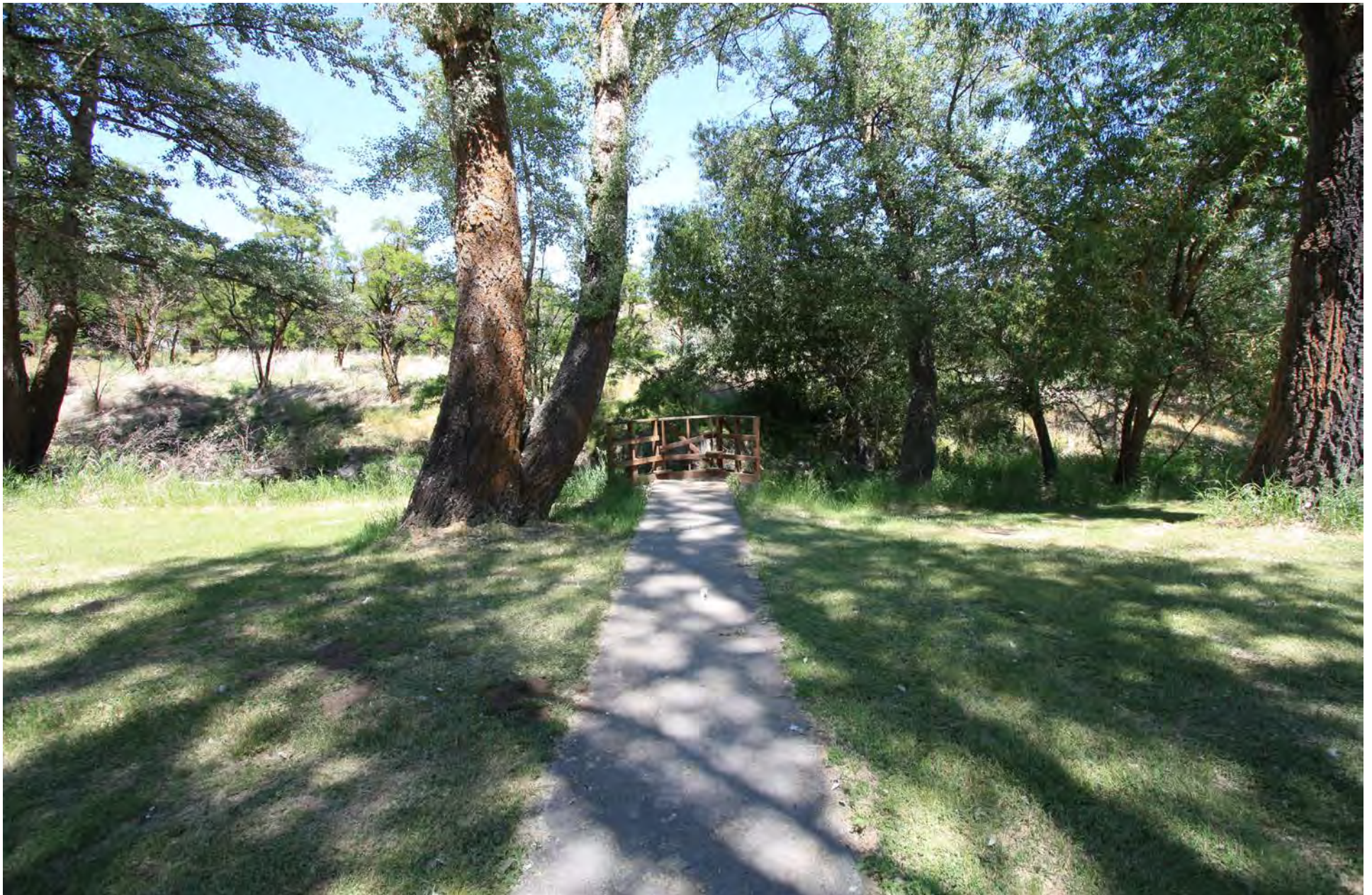
Photo 3. Bridge Remnants, contributing structure to NRHP listing. Looking N. 6/15/2018.
