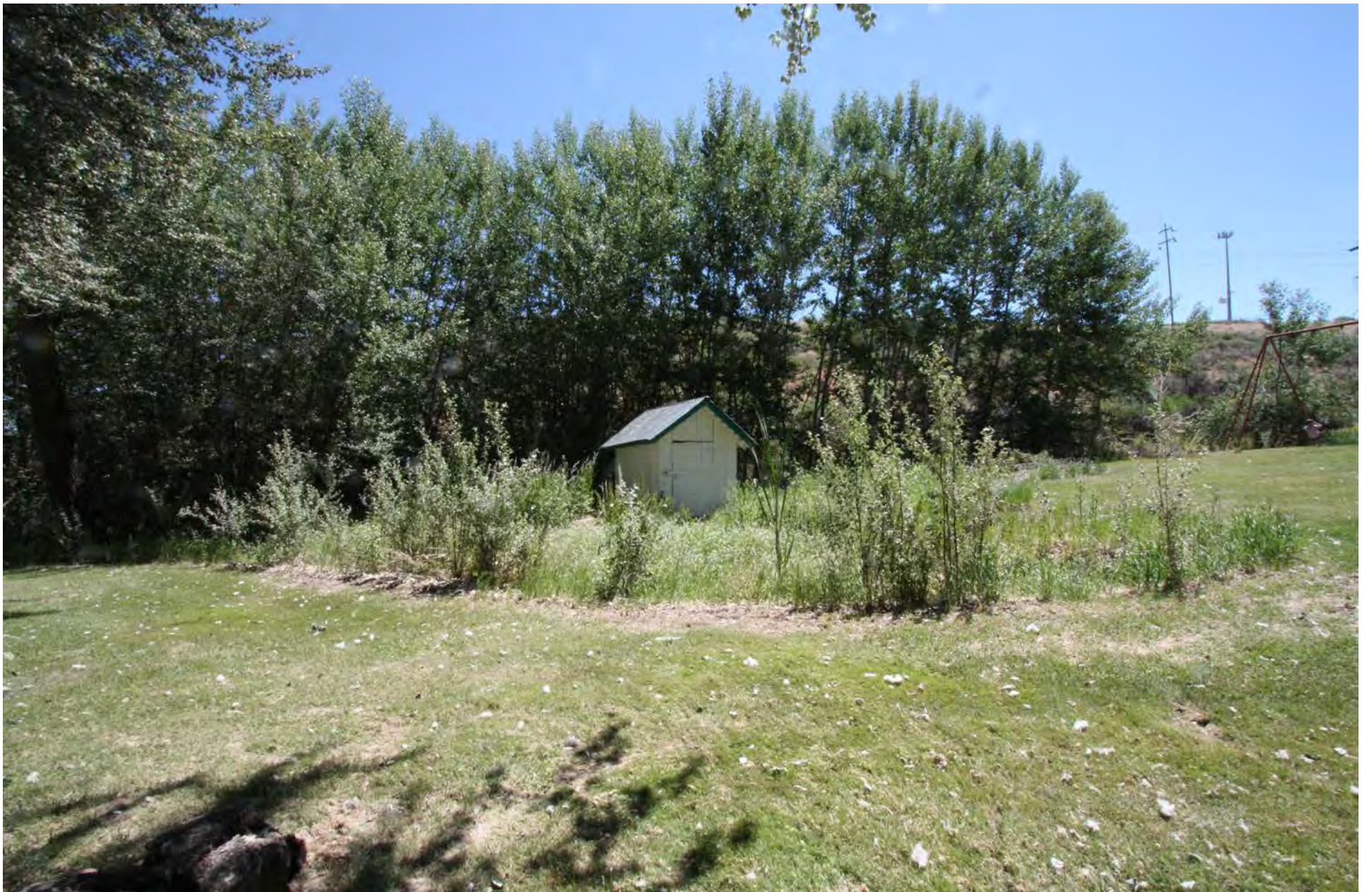
Photo 2. Pumphouse, contributing structure to NRHP listing. Looking E. 6/15/2018.
