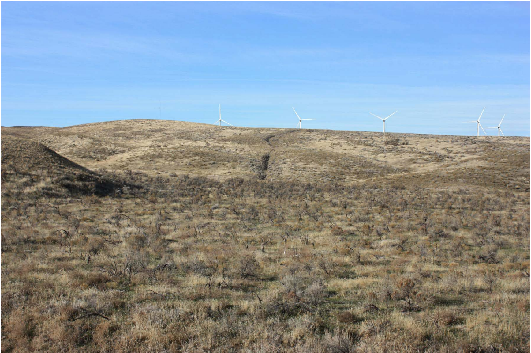
Looking West at the GE 3.0-MW Montague Turbines from the Fourmile Canyon BLM Interpretive Site.
