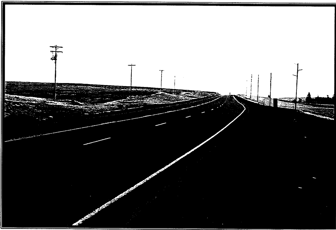
PHOTO R- 6: US 97 at MP 12 looking south.
