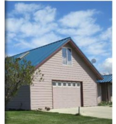
ody Ln., Stanfield, OR. View to the Northeast.
