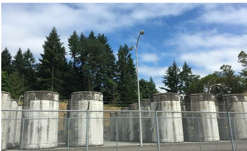
Trojan’s spent nuclear fuel is now stored in 34 passive-cooled containment vessels at the former plant site.
