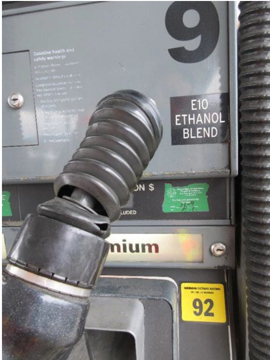
(AQGP-23) Balance System- bellows torn
