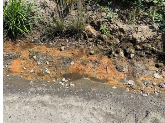
Close-up view of SEEP3 next to haul road (August 7, 2020).
