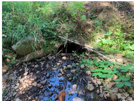
View of culvert below confluence of two drainages. (August 7, 2020)
