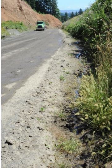
View of lower switch back of haul road and SEEP3 (July 16, 2020).
