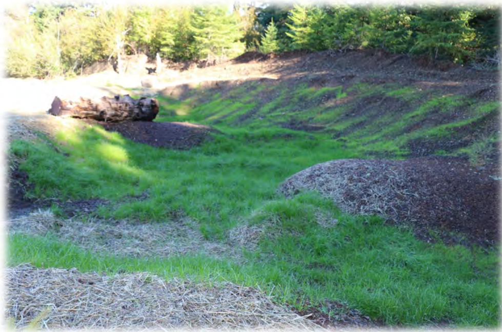
Dry Pond #3 with vegetated side slopes and bottom
