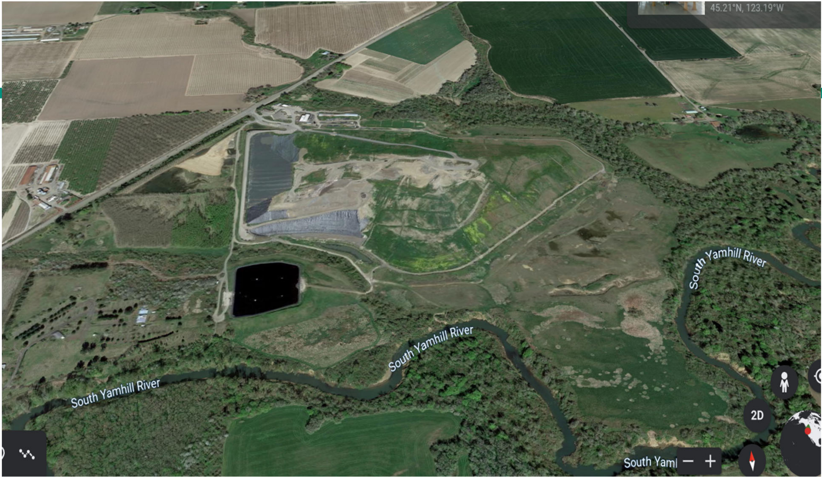
Aerial view of Riverbend Landfill
