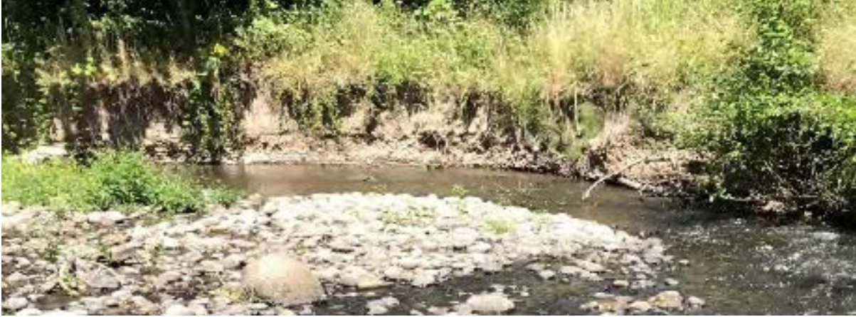
Figure 3a: Scarp at Johnson Creek Oxbow prior to temporary jute bag installation (Landau, 2017)
