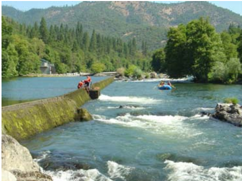
Gold Hill Diversion Dam removal
