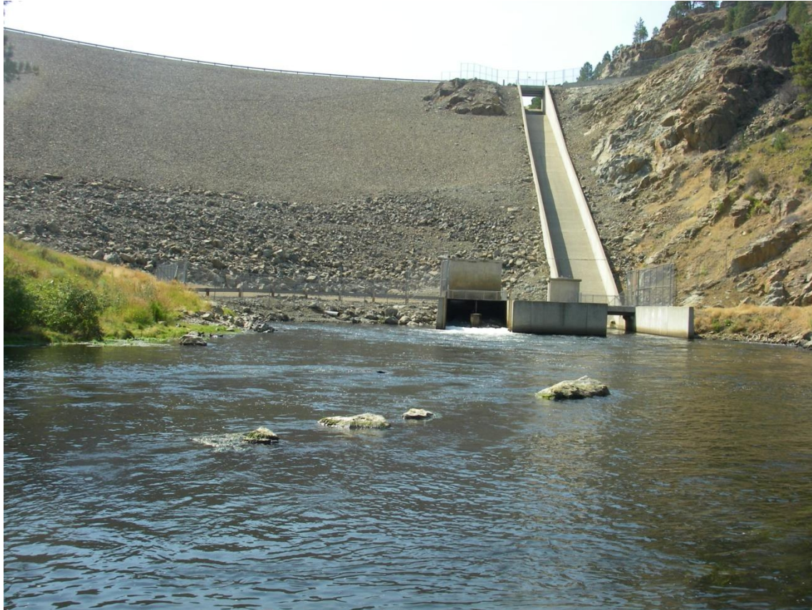
Figure 2: Mason Dam Spillway, Outlet Works, and Stilling Basin, August 2012.
