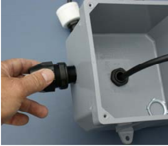
Install watertight Conduit connector.
