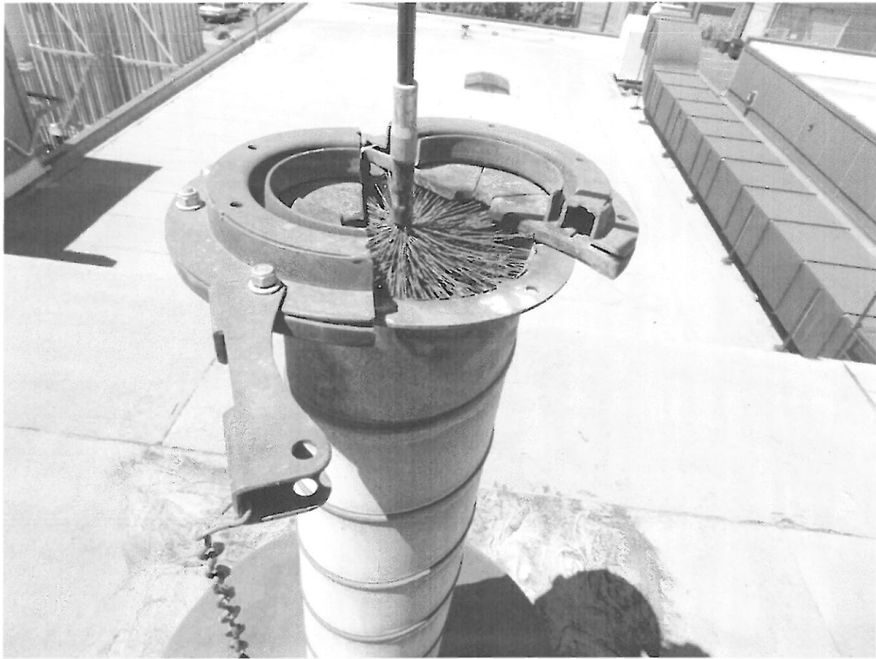
Cleaning cap installation
