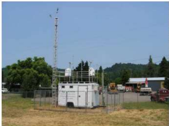
Oakridge WAC Air Monitoring Station.
