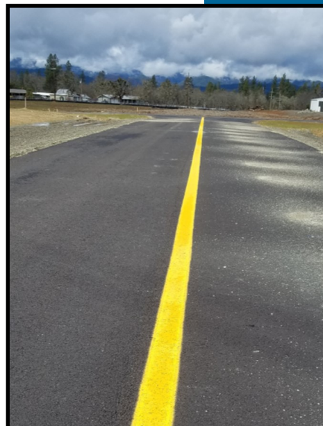
Grants Pass Airport: Parallel Taxiway Rehab Project 2018
