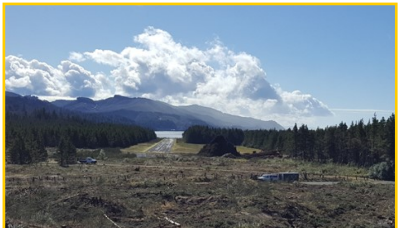
Nehalem Bay Obstruction Removal—after
