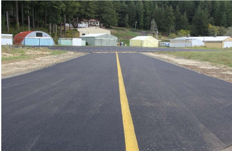
2020 - 2021: Ramp Paving ODAV SOAR Grant: $387,091
