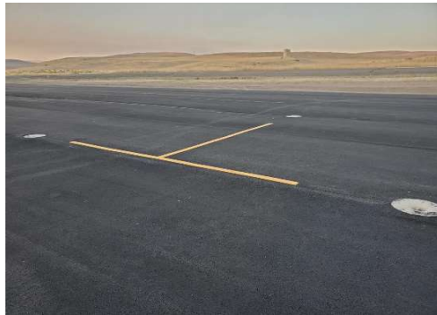
2021 - Tie-Down Area Improvements Project
