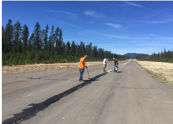
2016-2017: Minor Repairs to Runway ODAV SOAR Grant: $5,874
