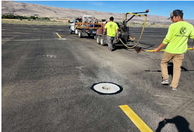
North Apron Reconstruction Total Project Cost: $1,939,144 ODAV COAR Grant: $150,000
