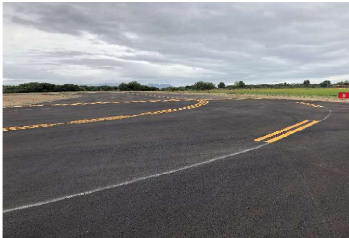
2019 - AIP 24: Taxiway A3 Realignment Project Total Project Cost: $3,520,285 ODAV COAR Grant: $150,000
