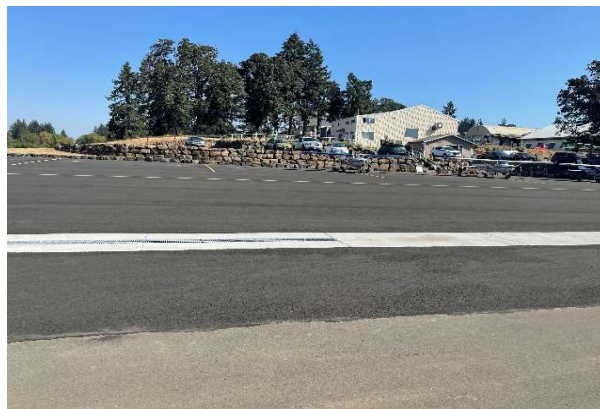
2021 - Transient Parking Ramp Total Project Cost: $188,900 ODAV COAR Grant: $94,450
