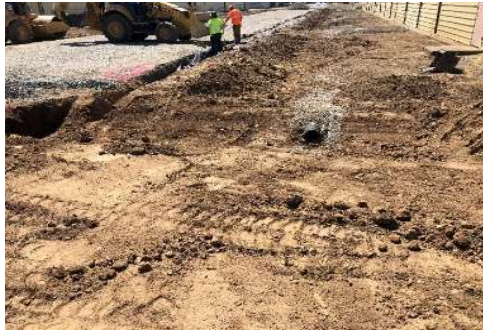
2019 - Taxiway Improvements Total Project Cost: $777,778 ODAV COAR Grant: $69,000
