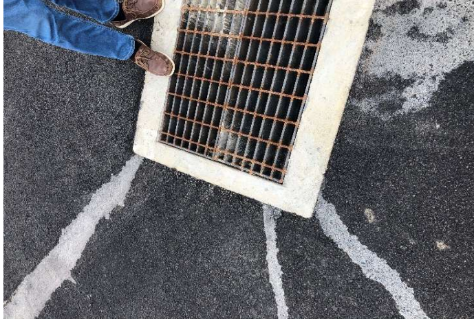
2019 - AIP 25: Ramp Rehabilitation Project Total Project Cost: $1,000,000 ODAV COAR Grant: $75,000
