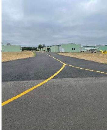
2021 - Runway Repaving Total Project Cost: $151,187 ODAV COAR Grant: $75,593.50
