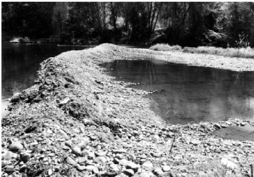
Push up dams have been used to divert water from Oregon streams since the 1800s. (Photo by Bob Brown/ Division of State Lands)
