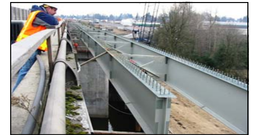
New steel bridge girders have been installed over the Columbia Slough
