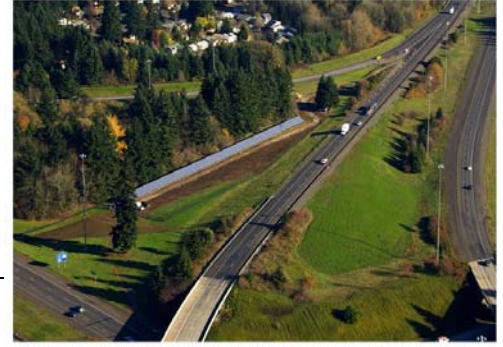
First solar highway project in Oregon and the nation.
