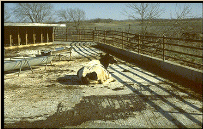
Concrete lots help contain wastes and keep animals out of the mud.
